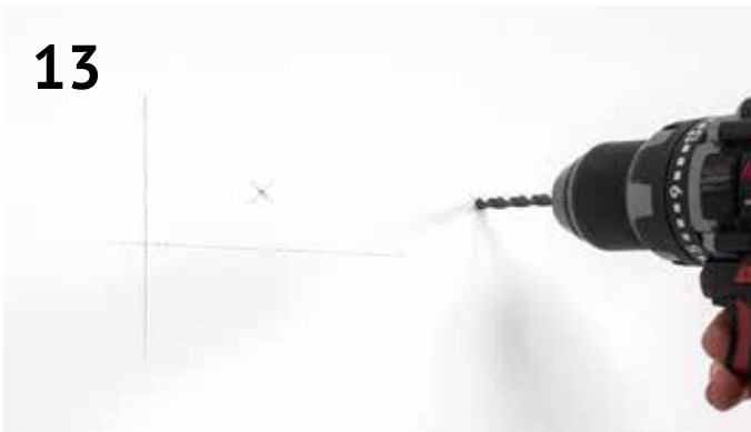
13 Drill the holes and install the 2 plugs
