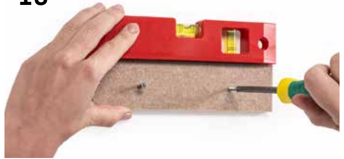
Position the felt spacer using a spirit level and screw in the second screw
