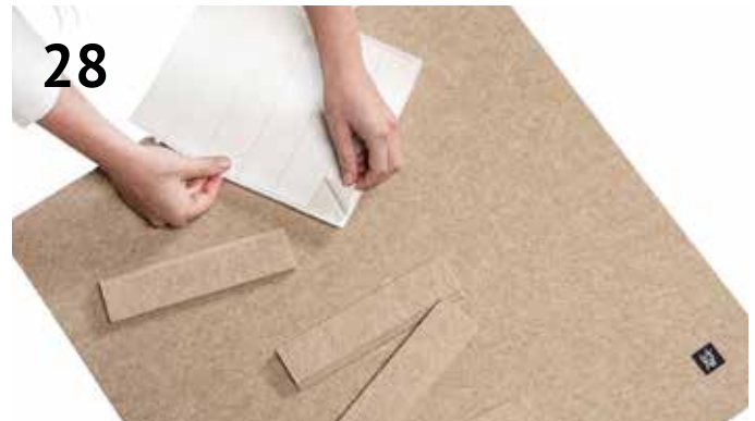
28 Option 2: Use double sided tape (enclosed sheets) Check the data sheet first
