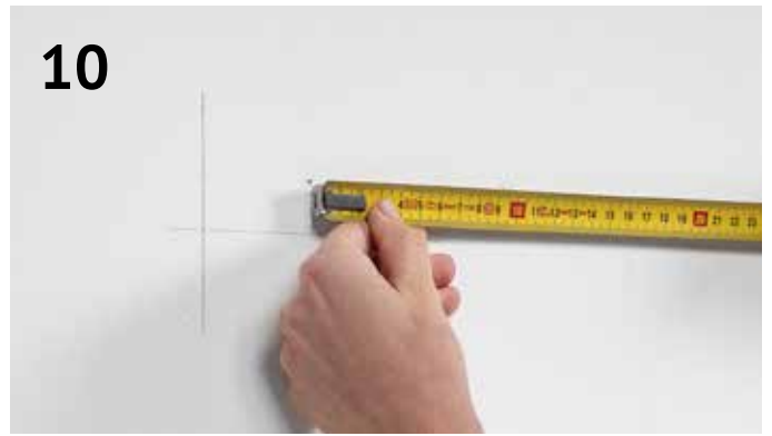
10 Measure a distance of 10 centimeters for the second drilling point
