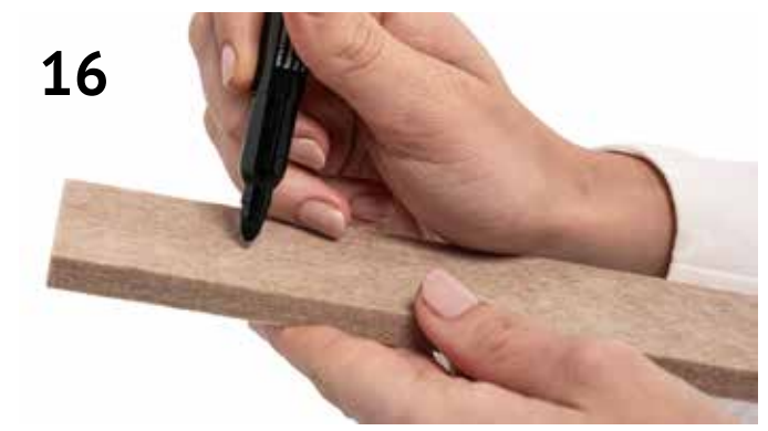
16 Use a marker to mark the drilling points on the felt spacer
