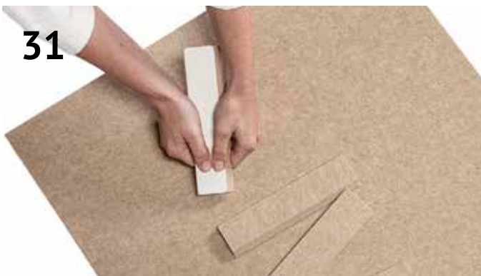
31 Keep pressing firmly for a few seconds to create a super strong bonding (!)
