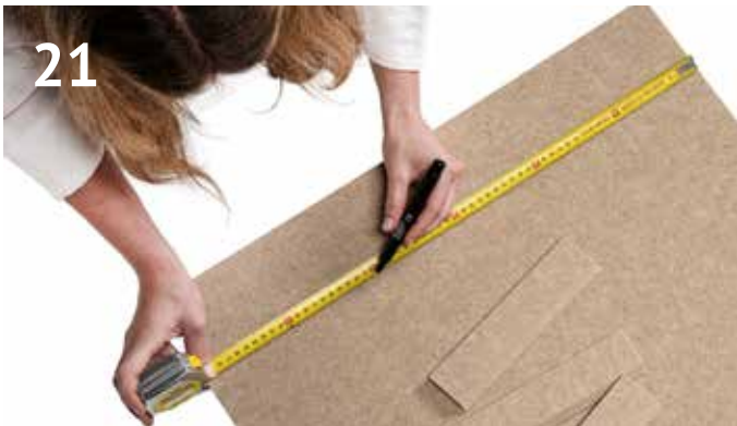
21 Check if the distance between the marked points is 20 centimeter (size of the felt spacer)
